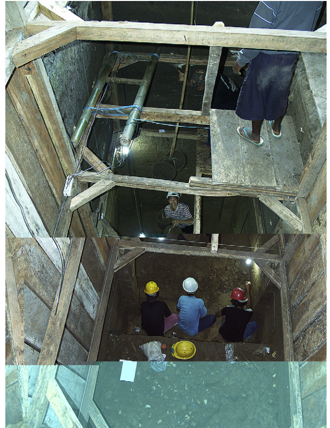
Figure 10. Our deep-trench excavations at Liang Bua relied on construction of wooden shoring and platforms as an essential safety measure (Photo: Djuna Iverigh).
